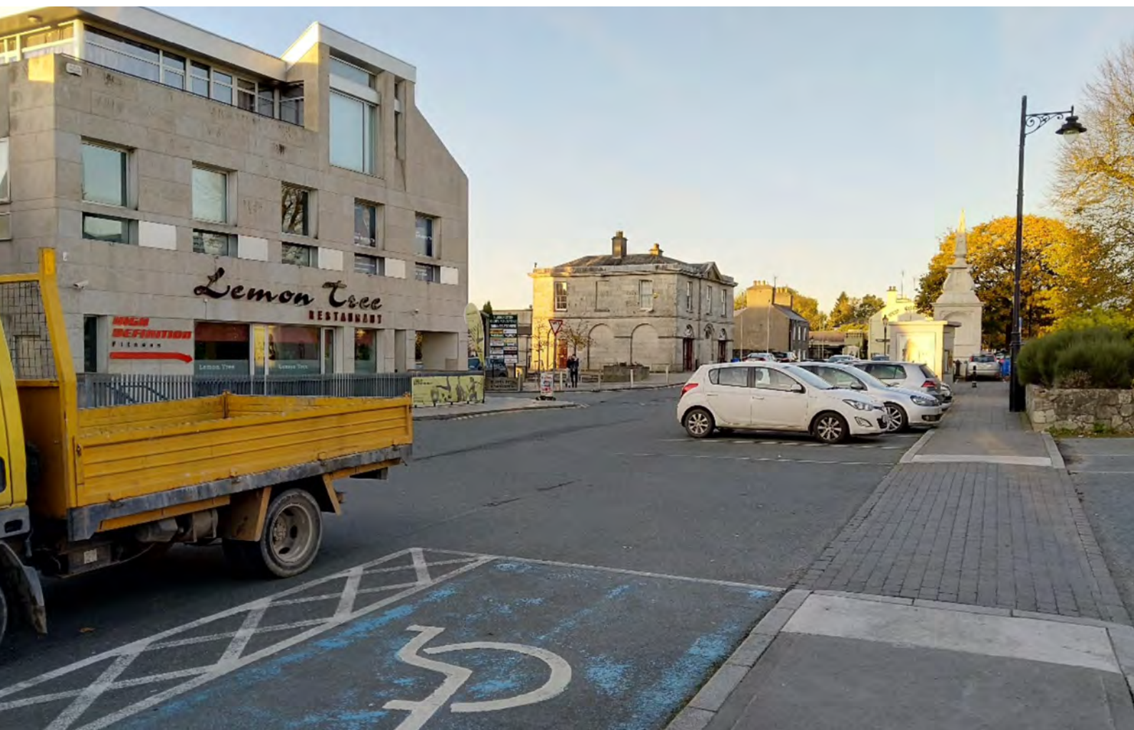
Figure 28 Focal points such as the Market Square prioritise car parking over pedestrian movement
